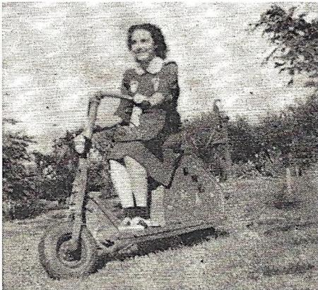
The attractive young lady in the picture above is riding a speedy motor scooter built by George W. Callard, R. F. D. 4, Albion, N. Y. It is powered with a Briggs & Stratton 1/2 h.p. motor and does 80 miles to the gallon of gas, Mr. Callard writes. Mr. Callard rates a \$3.00 Workbench check for his snapshot.
